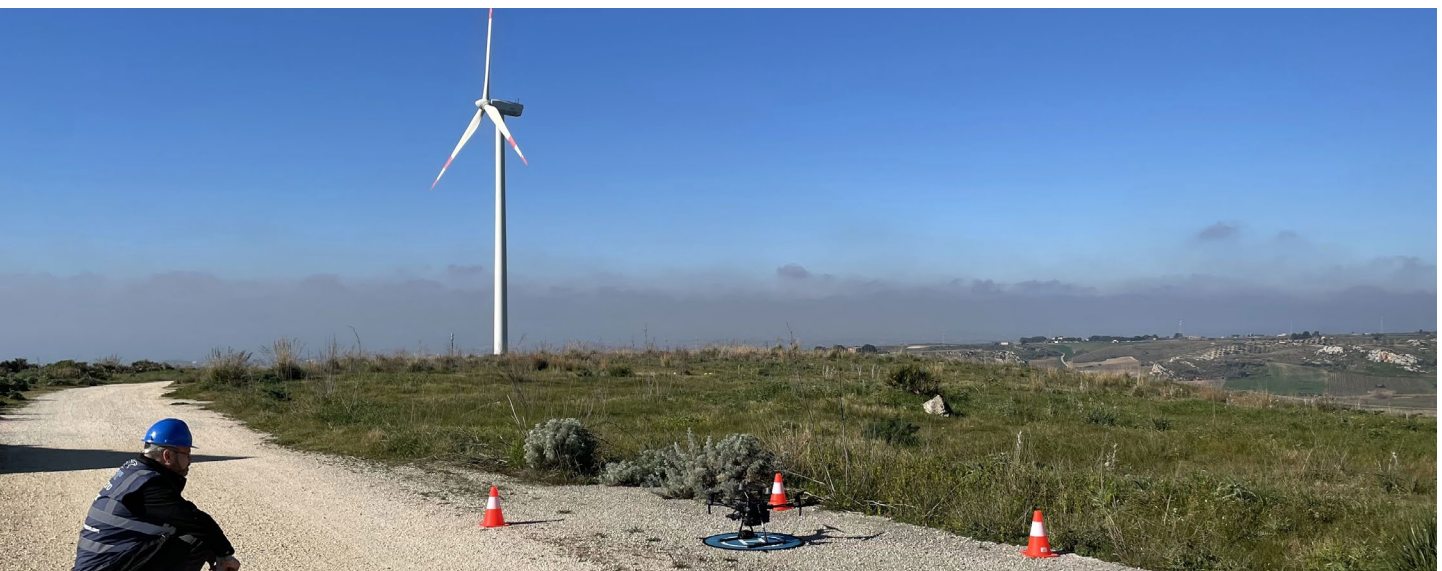
Inspection of wind turbine blades by drone - Lago Arancio plant - Italy
